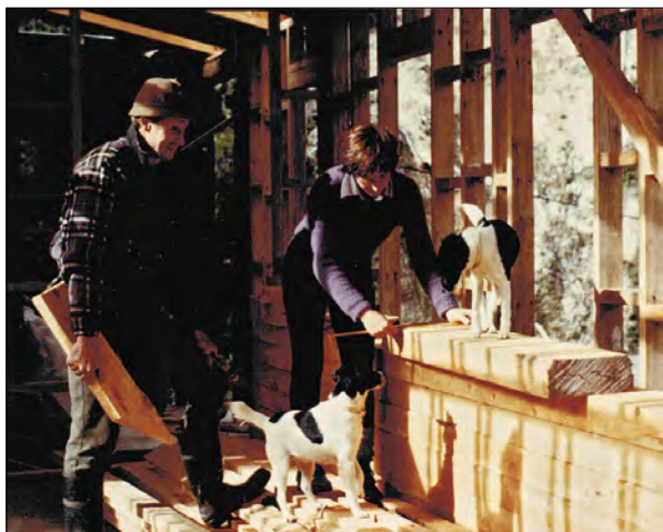
The window frames and door posts are all 8x4s that were milled at Staglands by Sarah. Here she is, left, checking the accuracy of her cutting with the help of her dogs
