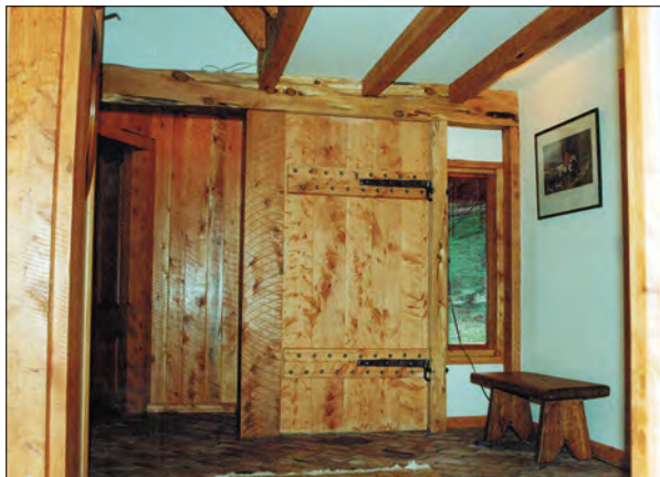
The front door of the house. I always like the look of heavy chunky timber, so we milled a truck-and-trailer load of macrocarpa logs into big beams and posts. I am often accused of over-building
